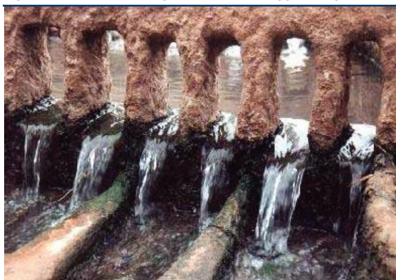
Figure 6.3 Water-Dividing Structure in a Foggara, Algeria
